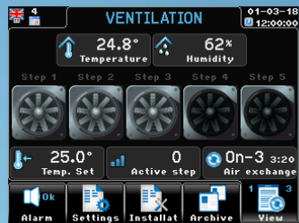
Viewing operating condition
