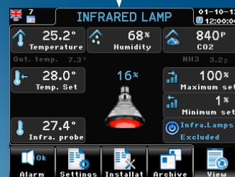
IR lamp heating view
